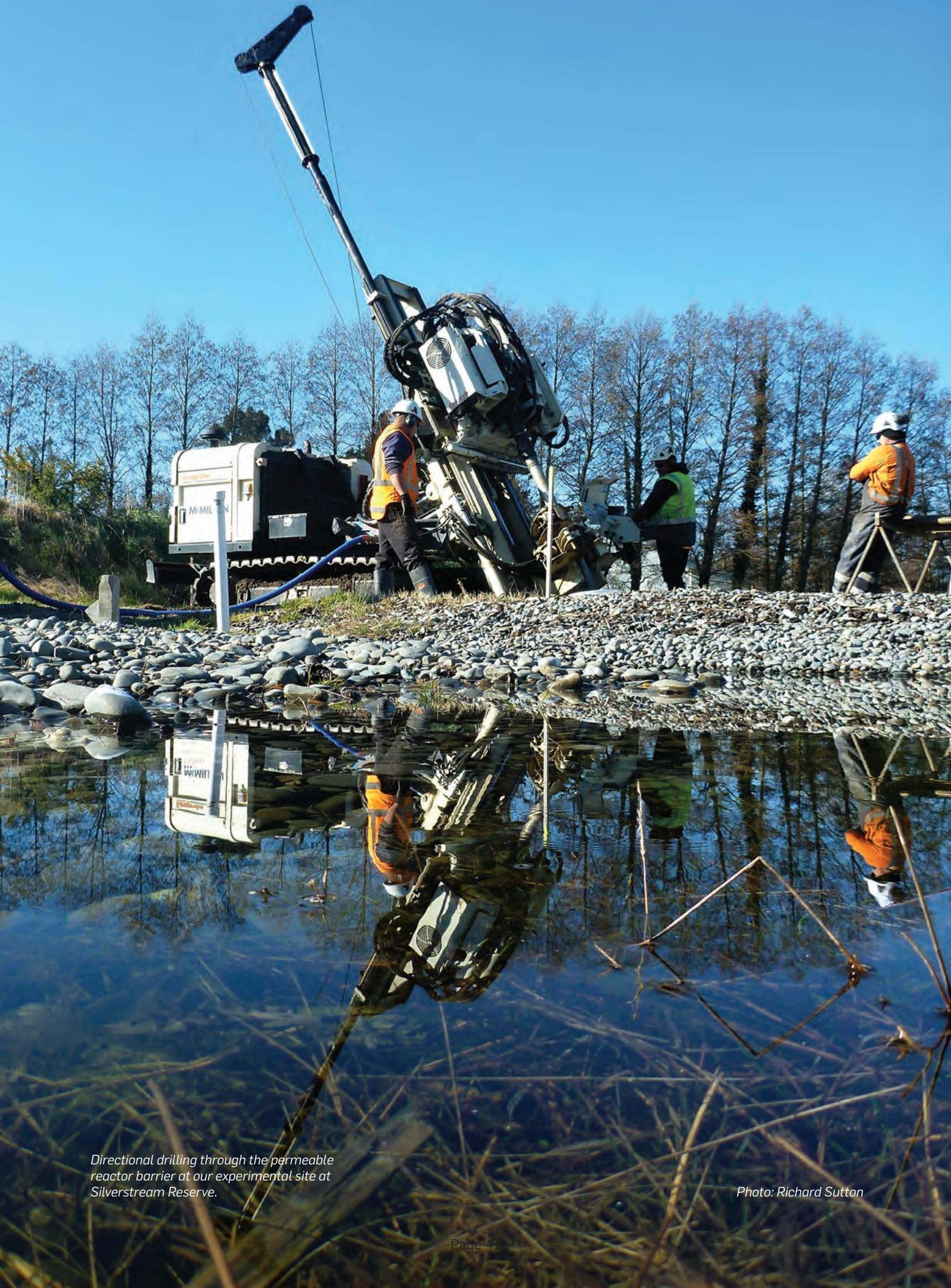
*Directional drilling through the permeable reactor barrier at our experimental site at Silverstream Reserve.*
